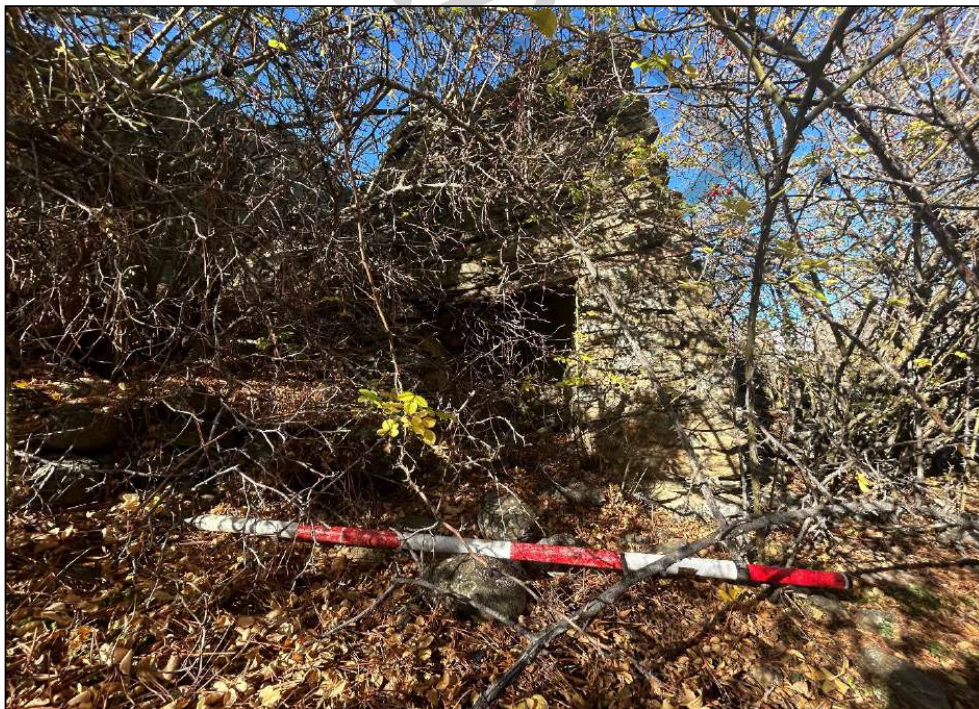
Figure 21. Base of fireplace, main portion of fireplace inaccessible due to briar, facing east.
