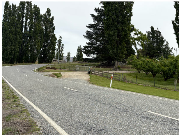
Figure 3: Photo of dual entranceway from Chapman Road
