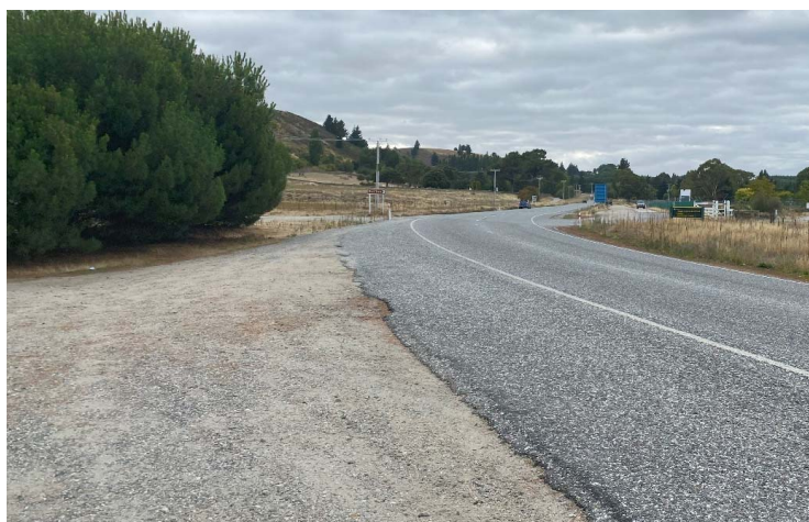
Photograph 3: Informal Access to Wide Road Reserve Looking East
