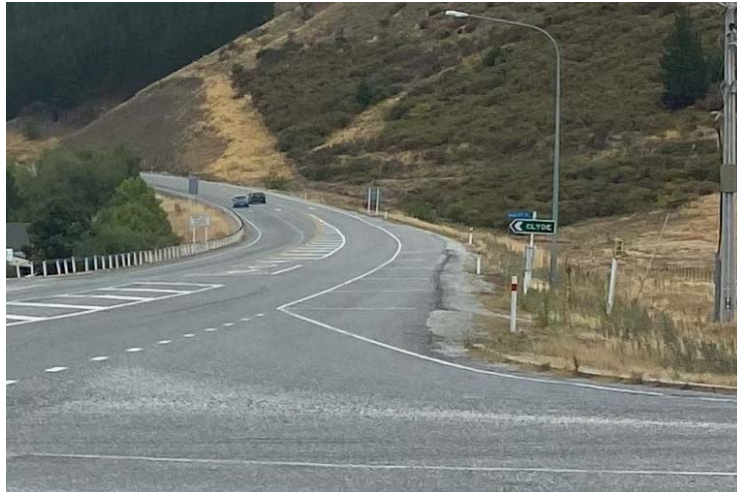
Photograph 5: Wide Shoulder on State Highway 8, North of Springvale Road
