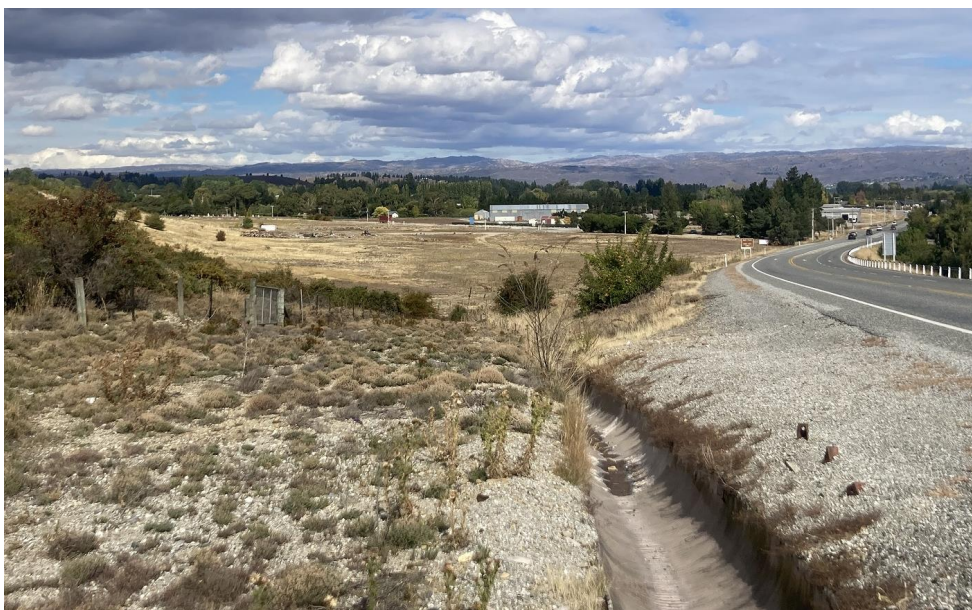
Photo 2. Looking southeast along the stormwater channel towards the development area beyond.
