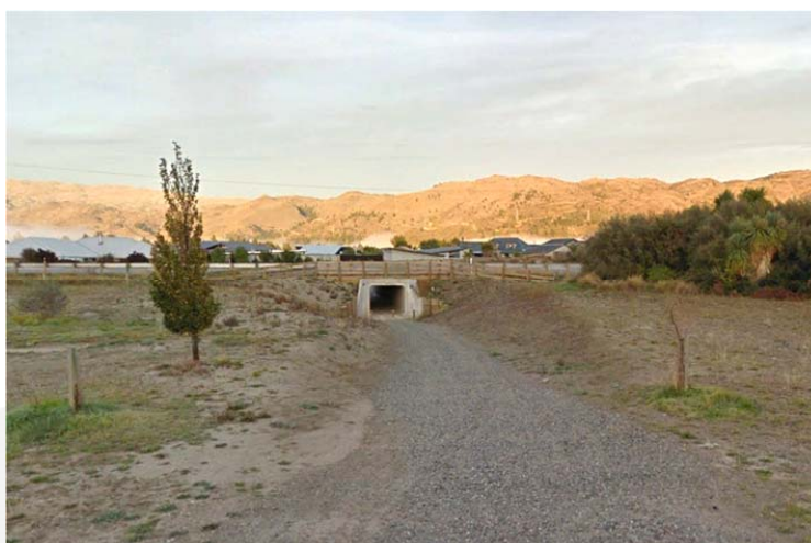
Photograph 7: Underpass below State Highway 8
