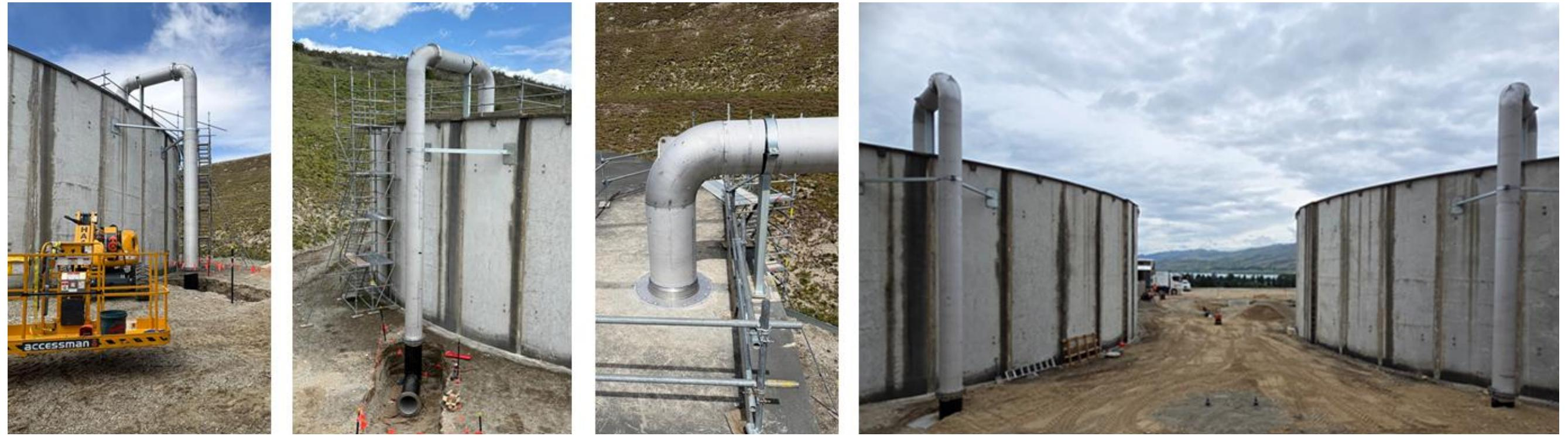
**Above – McNab Road reservoir site. New reservoir inlets constructed**
