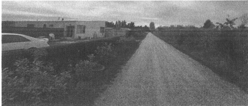
Figure 2: Weed matting along access easement (Source: Site visit 17 April 2025)
