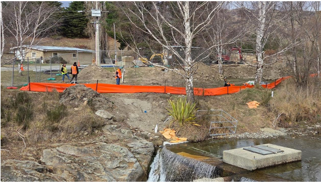
Above – Patearoa water treatment plant site. Water intake and pipeline works.
