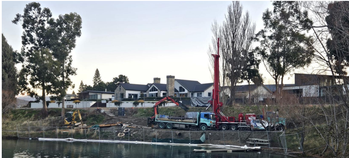
Above – left & right: Establishing of new bore between Lake Dunstan and Cromwell cycleway
