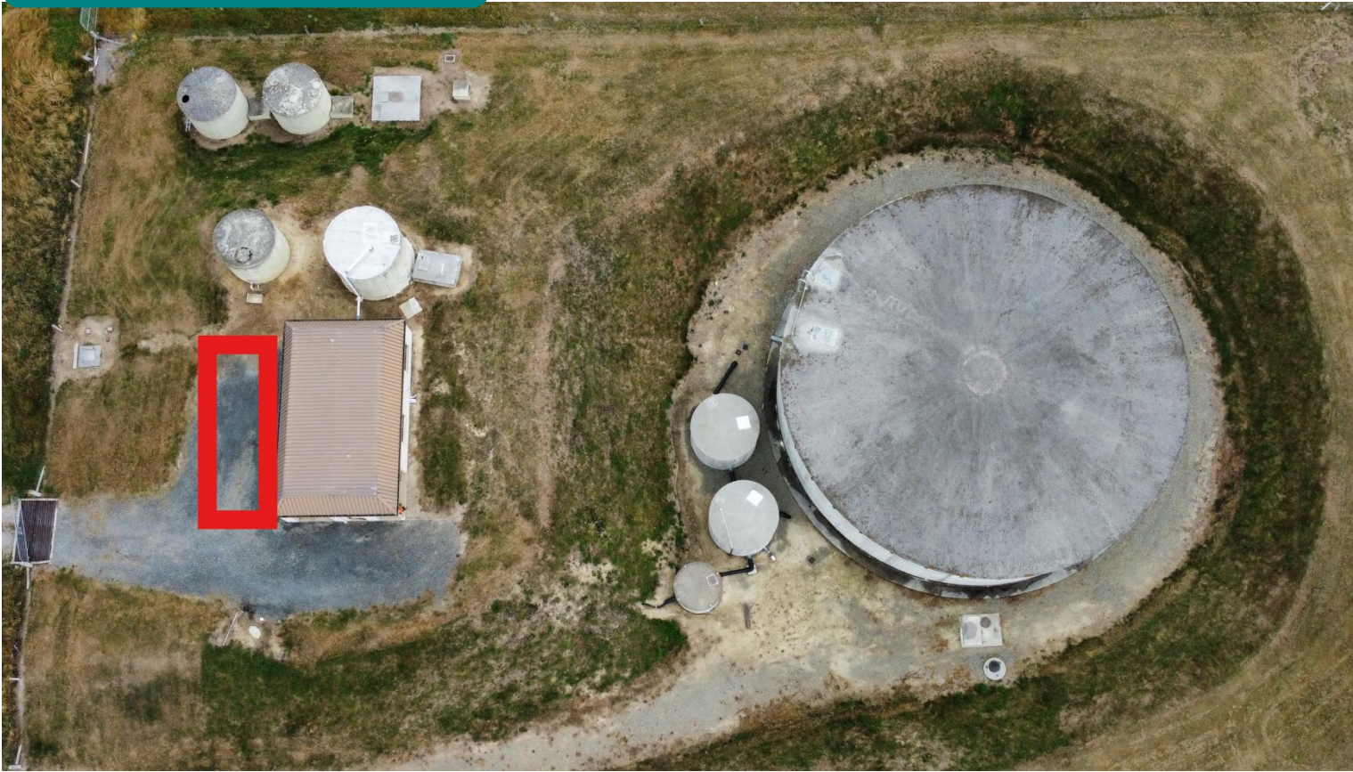
Above –Ranfurly water treatment plant site. Red box is where containerised water treatment plant will be installed.
