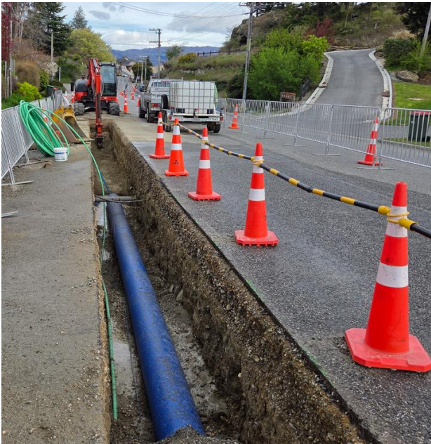
Installation of watermain Earnsclough Road
