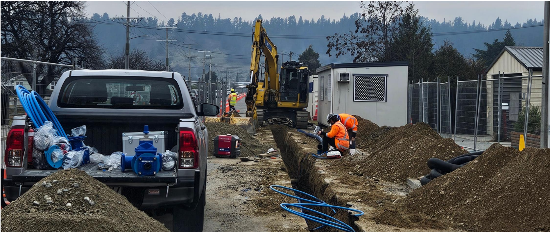
Above: Installation of watermain and laterals to property boundaries on Enterprise Street (opposite Dunstan High School)
