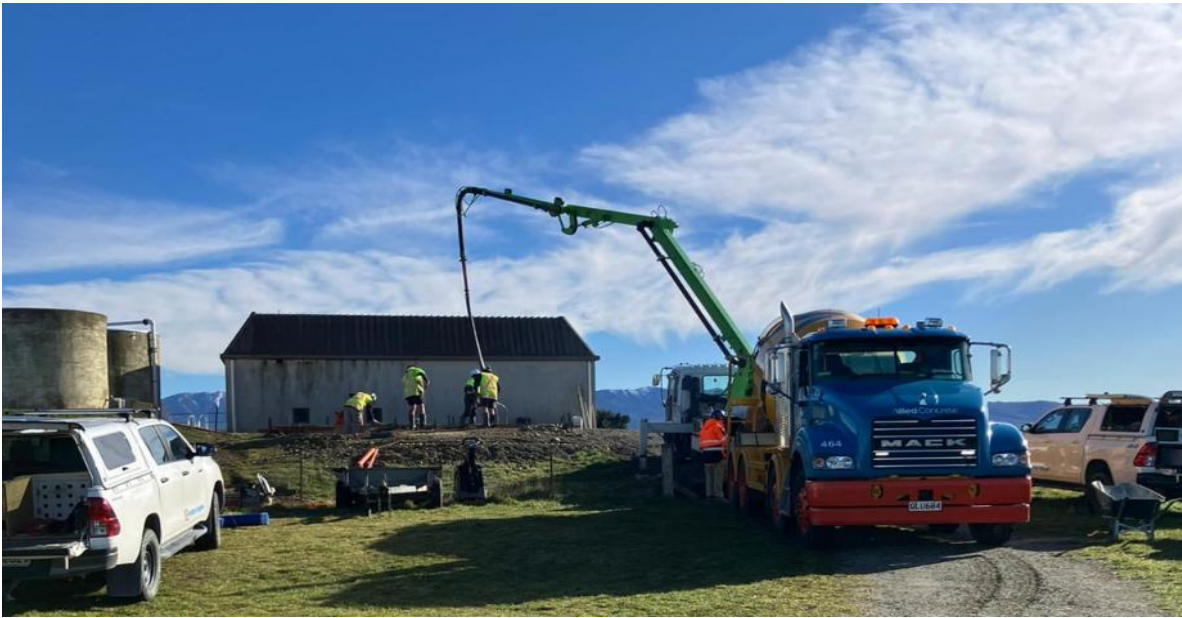
Above –Ranfurly water treatment plant site. Concrete building slab being poured
