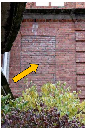
Fig. 299 Exterior image showing brick infill of original opening in the east elevation wall with flat segmental brick arch.
