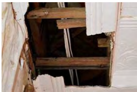
Fig. 190 Ceiling decay caused by water ingress in Space 1.31.
