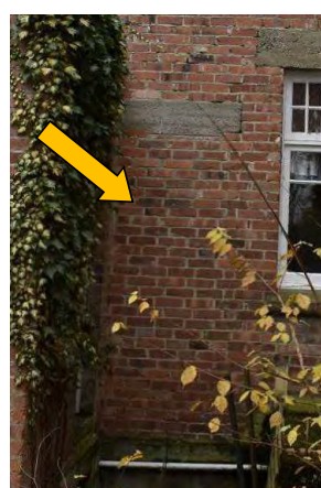
Fig. 349 Brick infill of original pantry window opening in the east elevation wall with concrete head lintel.
