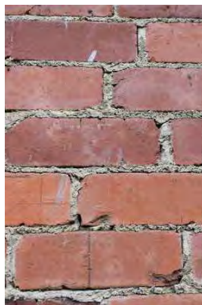
Fig. 32 Elevation typical brickwork without fair-faced finish.
