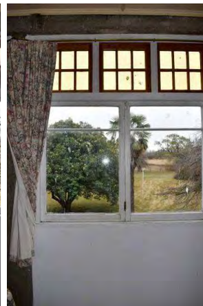
Fig. 156 Looking north across the Porch (Space 1.22). Note timber framed window units inserted between concrete columns and infill panel below window which covers the original balustrade.
