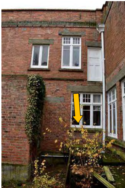
Fig. 344 Approximate location for the ash pit, noting that it was potentially incorporated under the floor slab as part of modification and relocation of the exterior wall.
