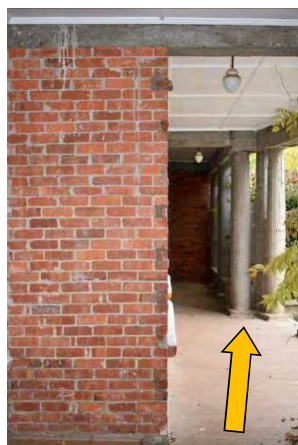
Fig. 307 Existing veranda columns which present either possible surviving fabric from the dividing wall installation or overspill from the original concrete pour.
