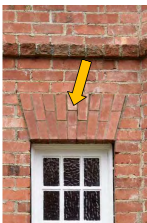
Fig. 268 Well struck pointing in the expressed brick flat segmental arch.
