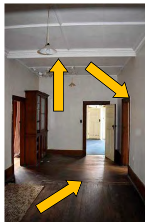
Fig. 326 Evidence of original wall alignment (arrowed).
