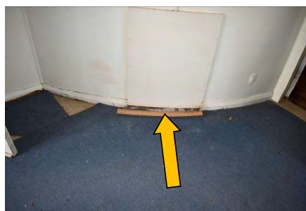
Fig. 341 Image showing the curved wall in Space 1.11 which conceals the original range alcove.
