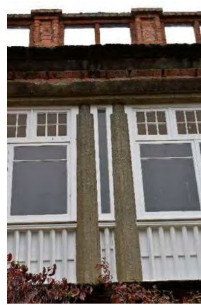
Fig. 21 Timber window joinery infill of the original balcony opening. Note the original concrete columns and timber balustrading remains legible.
