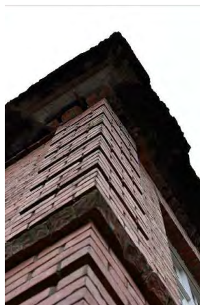
Fig. 52 Typical expressed brick quoins at first-floor level.
