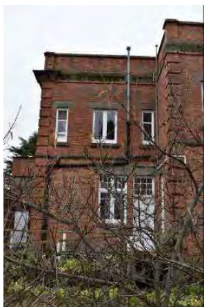
Fig. 25 Looking towards the west side of the south elevation. Note expressed brick quoins at all building corners, but more simply detailed concrete lintel window heads.
