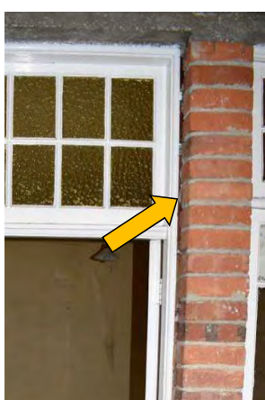
Fig. 269 Large gaps between the fenestration and brick reveals.
