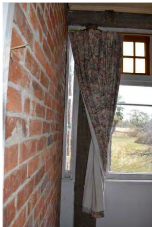
Fig. 154 Looking north across the Porch (Space 1.22). Note timber framed window units inserted between concrete column and dividing wall.
