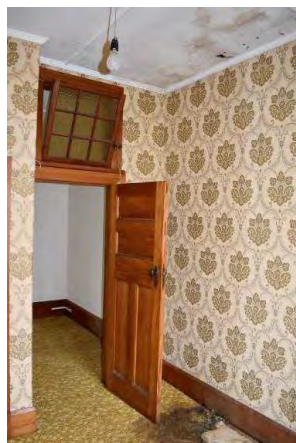
Fig. 361 Space 1.36 with evidence of water staining at ceiling, wall, and floor level.
