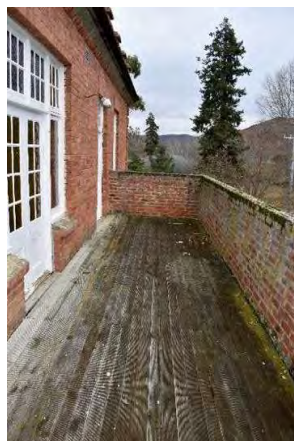
Fig. 296 West elevation veranda with concrete structure and brick masonry balcony balustrade.
