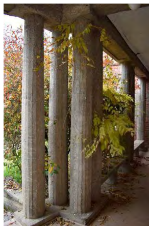
Fig. 60 Looking east through Space 1.01. Note the array of concrete columns supporting the two-storey veranda.
