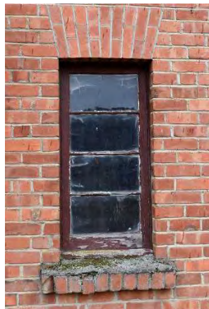
Fig. 376 Poor joinery finishes.
