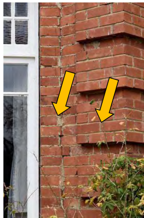
Fig. 358 Contrast between the generally poor wall pointing (left arrow) and well executed expressed brick elements (right arrow).
