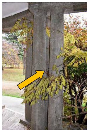
Fig. 308 Close-up view of existing veranda columns which present either possible surviving fabric from the dividing wall installation or overspill from the concrete pour.
