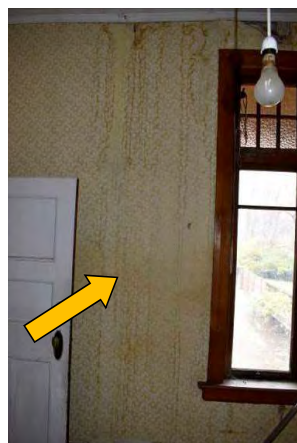
Fig. 330 Interior view showing the location of the blocked-up opening in the west elevation wall.
