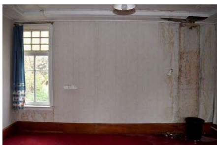
Fig. 188 Looking south across Space 1.31. Note wall staining and decay caused by water ingress.
