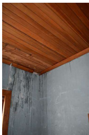
Fig. 219 Space 1.39. Note staining at wall and ceiling from water ingress.
