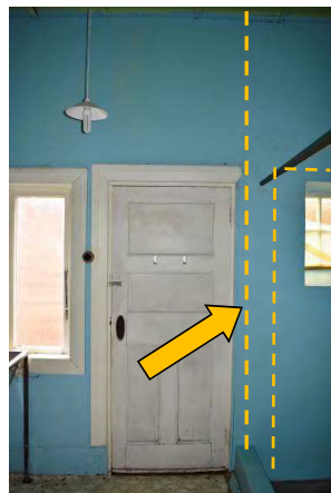
Fig. 334 Original alignment of the partition wall between the coal storage shed and the staff bathroom and the infilled doorway.
