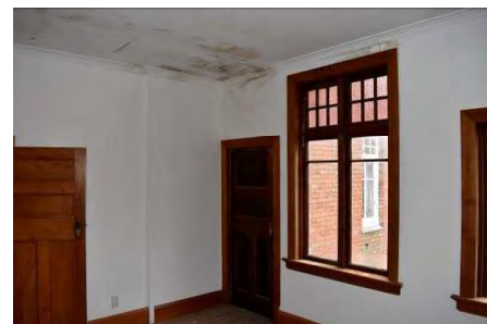
Fig. 209 Space 1.37 looking north-east. Note staining at ceiling level from water ingress.
