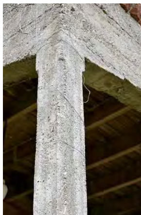
Fig. 49 Veranda concrete post and beam support structure. This structure has not been completed with the final render surface.
