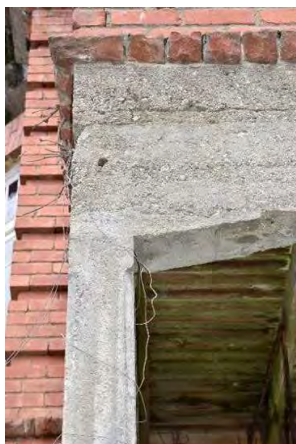
Fig. 50 Veranda concrete post and beam support structure. This structure has not been completed with the final render surface.
