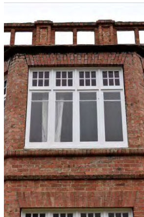
Fig. 17 Typical four-unit timber window joinery with multi-paned awning top light, and lower casement featuring single horizontal glazing bar in the upper portion of the opening.
