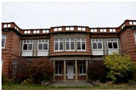
Fig. 291 North elevation with brick parapet and openings which were designed to hold the Roman lattice motif.
