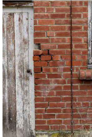
Fig. 371 Poor joinery finishes and loss of pointing mortar.
