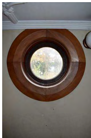
Fig. 71 Feature porthole window located within the south elevation at the staircase first landing. Note modified ceiling cutting through the window architrave.
