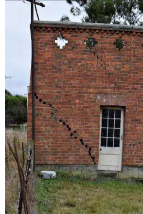
Fig. 372 Significant cracking in the brick masonry from foundation settlement.
