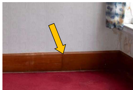
Fig. 323 Close-up view of scarfed-in timber skirting.
