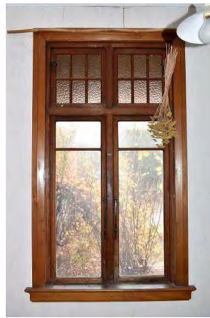
Fig. 106 Typical two-unit timber window joinery with multi-paned awning top light, and lower casement featuring single horizontal glazing bar in the upper portion of the opening.
