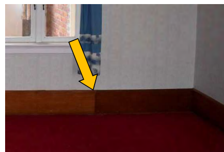
Fig. 319 Evidence of alterations to the wall in this location with a scarfed-int timber skirting which is different in finish to that evident elsewhere in the Sunroom.
