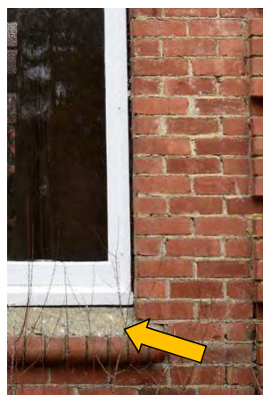
Fig. 272 Rough concrete finish to the sill which requires a render finish to complete the profile.
