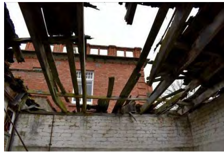
Fig. 135 Looking at Space 1.16. Note dilapidated ceiling and roof fabric.
