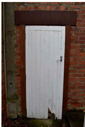
Fig. 139 Timber tongue and grooved entrance door for Space 1.18.
