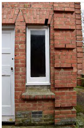
Fig. 46 Looking towards the original staff bathroom door and window. Note typical expressed brick flat segmental arch over door and window openings, and the expressed brickwork quoins at the building corner.
