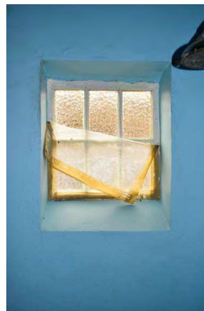
Fig. 335 The non-original window fitted into the door opening brick infill.
