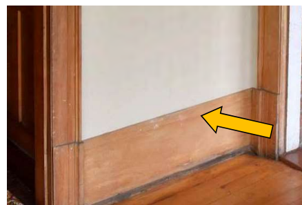
Fig. 317 Evidence of alterations to the wall with a different profiled skirting to elsewhere in the Sunroom.
