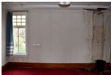
Fig. 365 Space 1.31 with evidence of water staining at ceiling, wall, and floor level.
