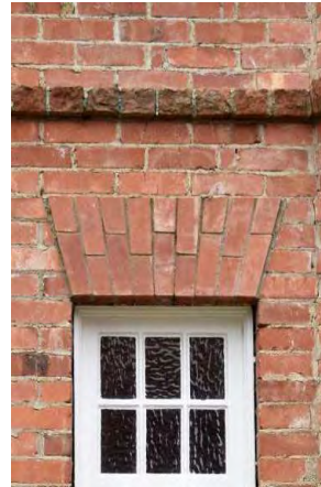
Fig. 18 Typical window with flat segmental brick arch over the window opening.
