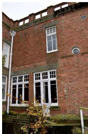
Fig. 27 Looking towards the central portion of the south elevation. The elevation features typical window joinery with multi-paned awning top light, and lower casement featuring single horizontal glazing bar in the upper portion of the opening. Note the feature porthole style window.
