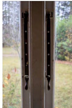
Fig. 90 Typical window ironmongery in Space 1.06.
