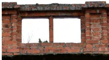
Fig. 292 The brick parapet and large openings which were designed to hold the Roman lattice motif.
