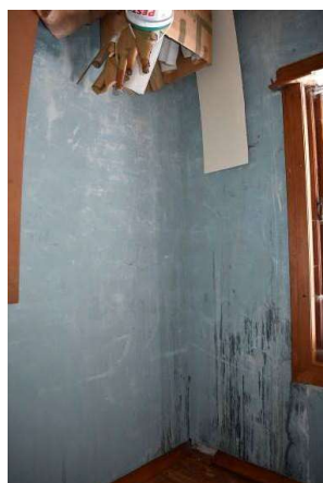
Fig. 218 Space 1.39. Note staining on wall from water ingress.
