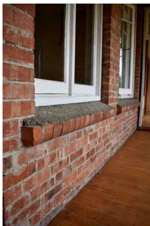
Fig. 146 South wall of the Sunroom (Space 1.21). Note brickwork is not fair-faced and awaits render finish.
