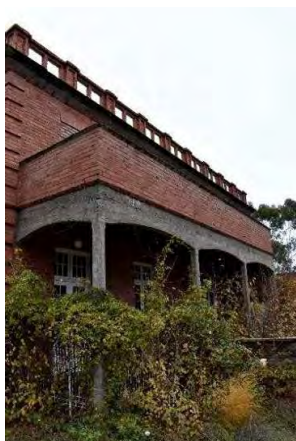
Fig. 295 West elevation veranda with concrete structure and brick masonry balcony balustrade.
