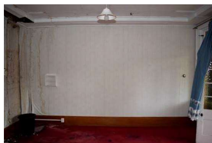
Fig. 189 Space 1.31. Note wall staining and decay caused by water ingress.
