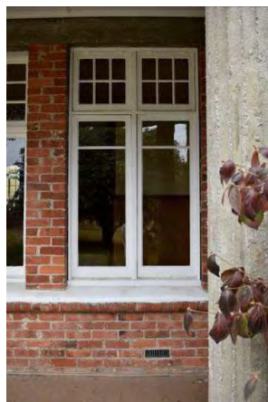
Fig. 65 Space 1.01 with typical two-unit timber window joinery with multi-paned awning top light, and lower casement featuring single horizontal glazing bar in the upper portion of the opening.
