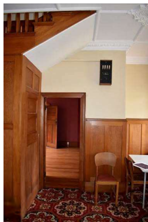
Fig. 70 Looking west from Space 1.02. Note oak wainscoting panels lining the entrance hall walls.
