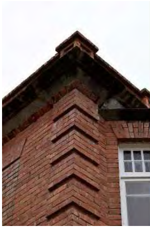
Fig. 19 Exposed brickwork quoins at corner of the projecting wings.
