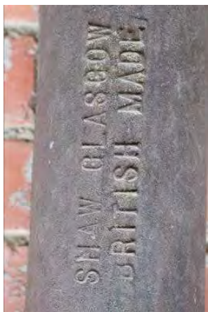
Fig. 31 Cast-iron foul water disposal pipework with manufacturer's stamp.
