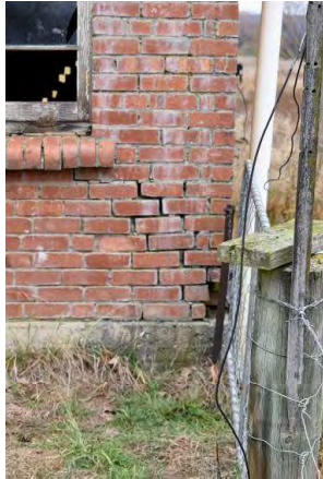
Fig. 370 Significant cracking in the brick masonry from foundation settlement.
