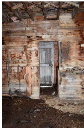
Fig. 377 Interior of the Stable Block and extent of moisture ingress.
