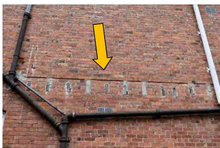
Fig. 284 Location on south elevation at first-floor level where the balcony was installed. Note the embedded timber joist off-cuts.
