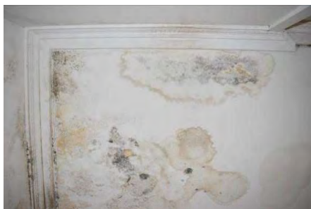
Fig. 366 Space 1.37 showing staining on ceiling from water ingress.
