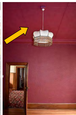
Fig. 309 Dining Room ceiling does not feature the elaborate plaster detailing as evident in other spaces of similar status. This may indicate that the ceiling was altered following the secondary staircase modifications.
