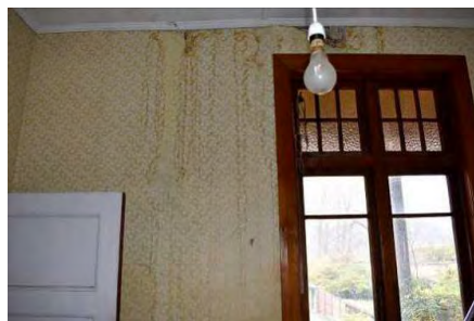
Fig. 367 Space 1.10 showing staining on ceiling and walls from water ingress.
