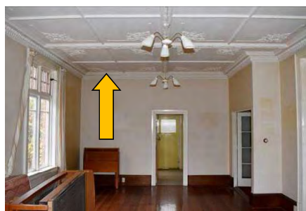
Fig. 306 Billiard Room which does not feature a fireplace in the location shown on the original plans. Also note the decorative ceiling pattern and cornice is consistent throughout with no infill repair evident.
