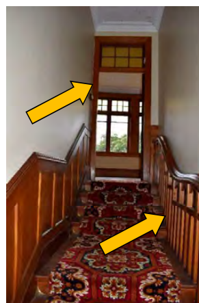
Fig. 313 Expressed handrail and balusters on right of stair would suggest that the stair originally opened into a double-height entrance hall space. Also note the doorway is not centrally placed in wall at the top of the stairs.
