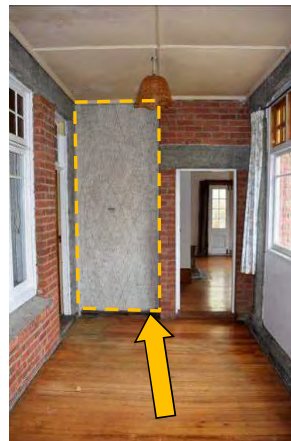
Fig. 355 Infill of original recess in the east elevation wall.
