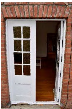
Fig. 54 Typical original timber door joinery with multi-paned doors.
