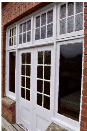
Fig. 53 Typical original timber door joinery with multi-paned top lights and doors.
