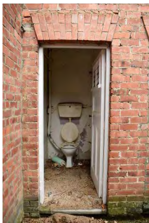
Fig. 44 Looking towards the original staff toilet. Note typical expressed brick flat segmental arch over door opening.
