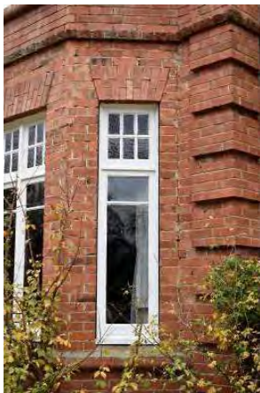
Fig. 16 Typical timber window joinery with single-unit, multi-paned awning top light, and lower casement featuring single horizontal glazing bar in the upper portion of the opening.
