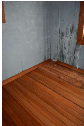
Fig. 362 Space 1.39 with evidence of water staining at ceiling, wall, and floor level.
