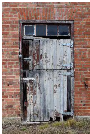
Fig. 375 Poor joinery finishes.
