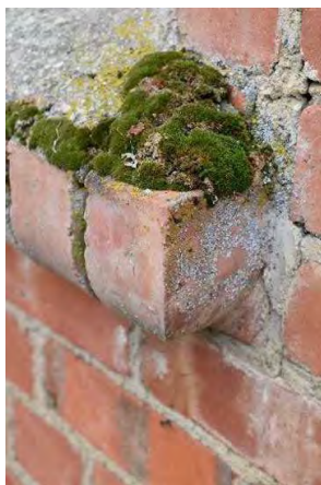
Fig. 51 Typical window-sill detailing featuring bull-nosed brickwork.
