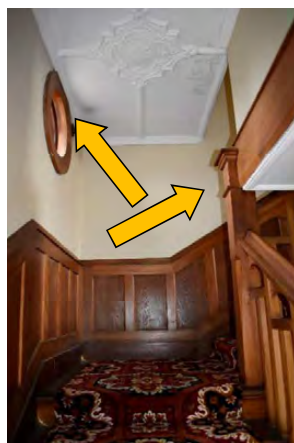
Fig. 312 Poor alignment of ceiling with window opening and newel post with floor structure.
