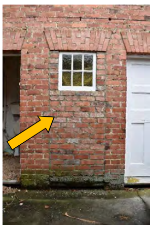
Fig. 333 Original coal shed doorway with brick infill and fitted window. The original flat segmented arch remains.
