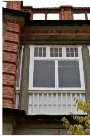
Fig. 20 Timber window joinery infill of the original balcony opening. Note the original concrete columns and timber balustrading remains legible. Note the timber balustrades are arranged in a diamond pattern on plan.
