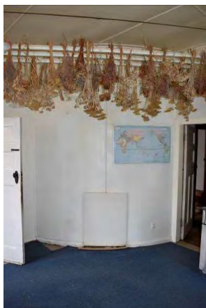
Fig. 116 Looking towards the curved wall in the north-west corner of Space 1.11. This wall conceals the original space containing the kitchen range.
