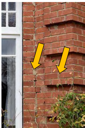
Fig. 265 Contrast between the generally poor wall pointing (left arrow) and well executed expressed brick elements (right arrow).
