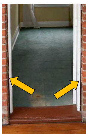
Fig. 270 Large gaps between the fenestration and brick reveals.
