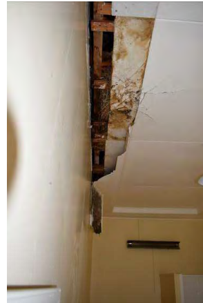
Fig. 179 Ceiling damage caused by water ingress within Space 1.27.
