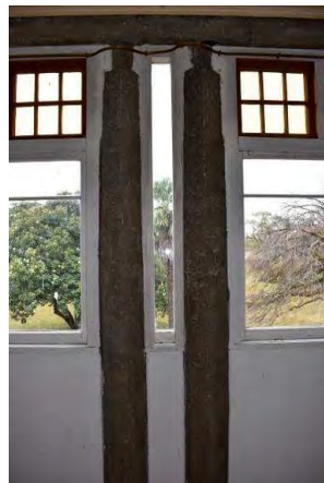
Fig. 155 Looking north across the Porch (Space 1.22). Note timber framed window units inserted between concrete columns
