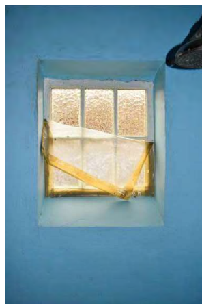
Fig. 119 Non-original window fitted within the original blocked-up door opening.
