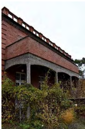
Fig. 41 Original veranda with concrete column and beam support structure and brick balustrade for the balcony
