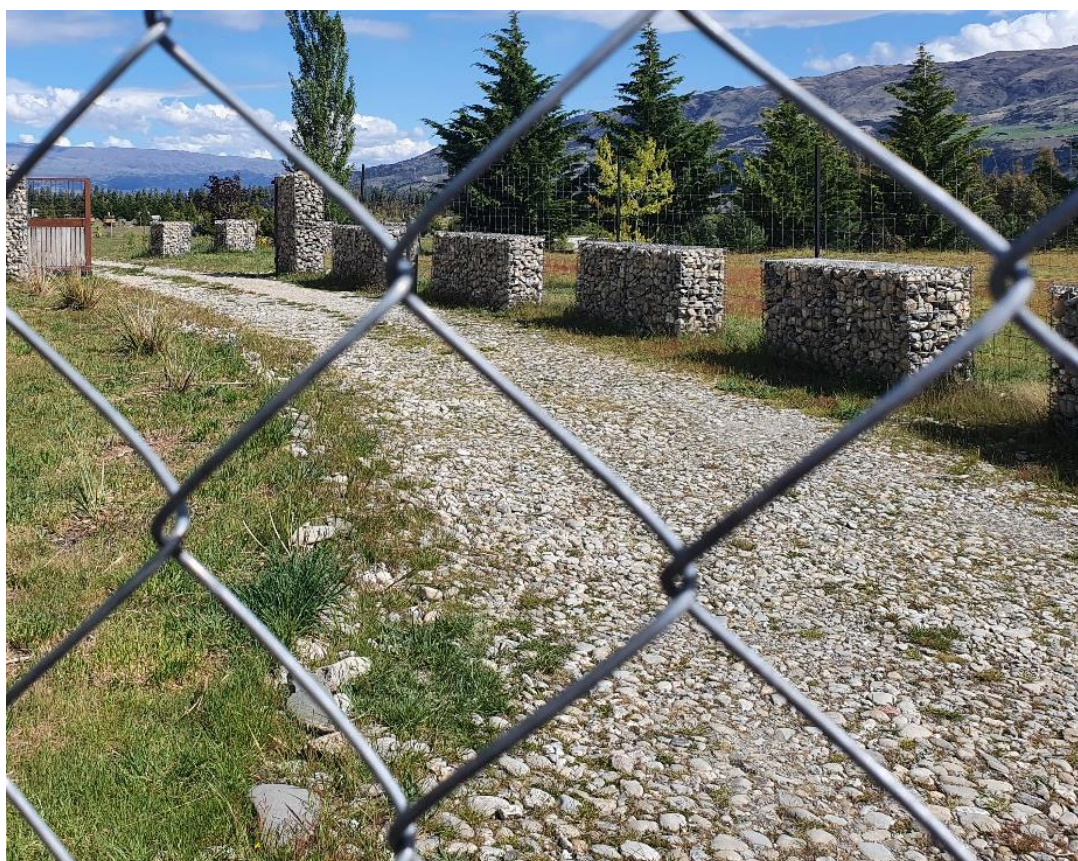
Figure Three: Photo from the north of the site looking into the double gate area. The fencing along the far side, behind the rock baskets, does not appear to have chicken wire along its base.
