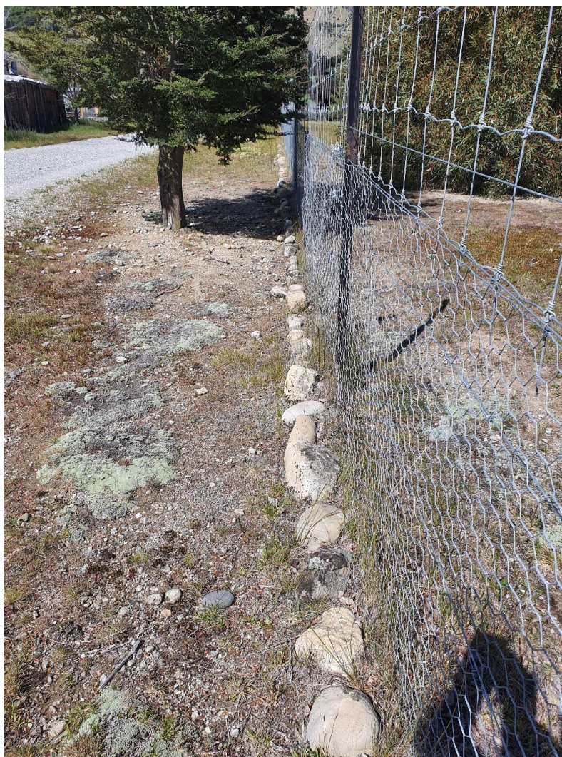
Figure One: Photograph of the boundary fence of the site along the northern boundary showing the line of rocks holding down the base of the fence. The applicant's property is to the right of the fence in this photo.
