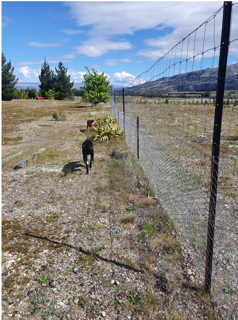
Figure Two: The fencing along the western boundary of the site, showing the provision of waratahs of differing heights along its length. Note that there are no weights on the base of the fence in this location. It appears to be simply bent over into the site.
