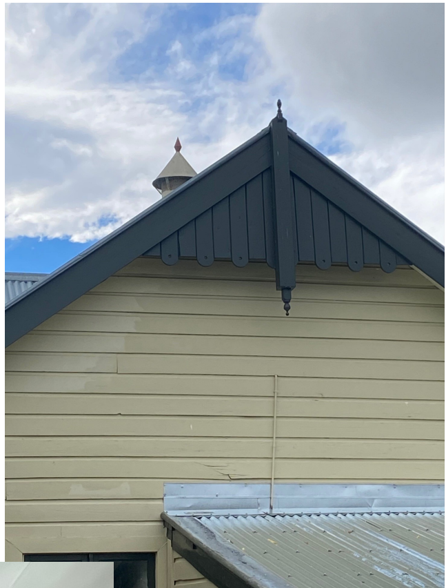
Refurbished roof apex detail and paint
