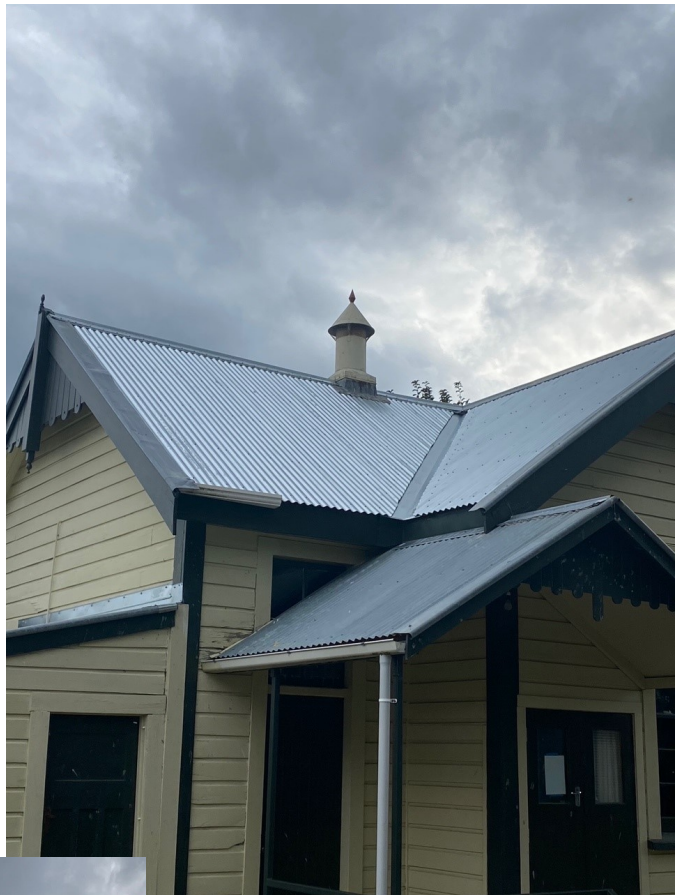
The roof with new roofing iron.
