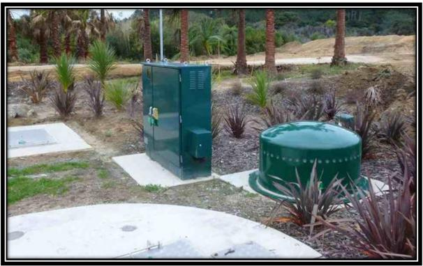
Figure 2 – Example of completed pumping station with landscaping
