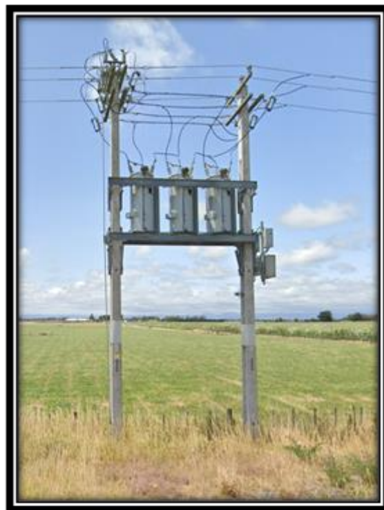
Figure 4 – Example dual poles with voltage regulators
