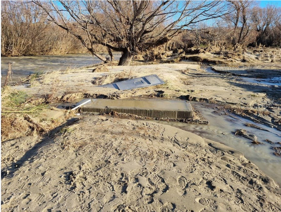
Effluent outlet structure – outlet blocked
