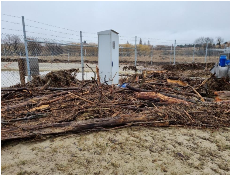
Debris around the influent point, screen and switchboard cabinet
