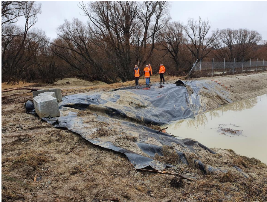
Pond 1 – Damaged section of liner pulled back into place and anchored
