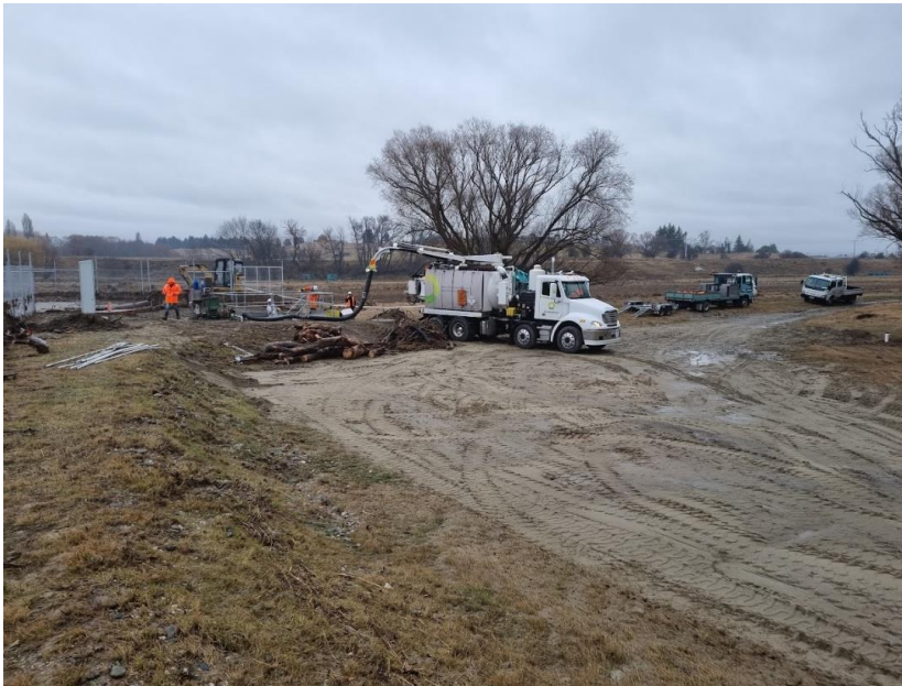
Jetting/cleaning of inlet screen chamber
