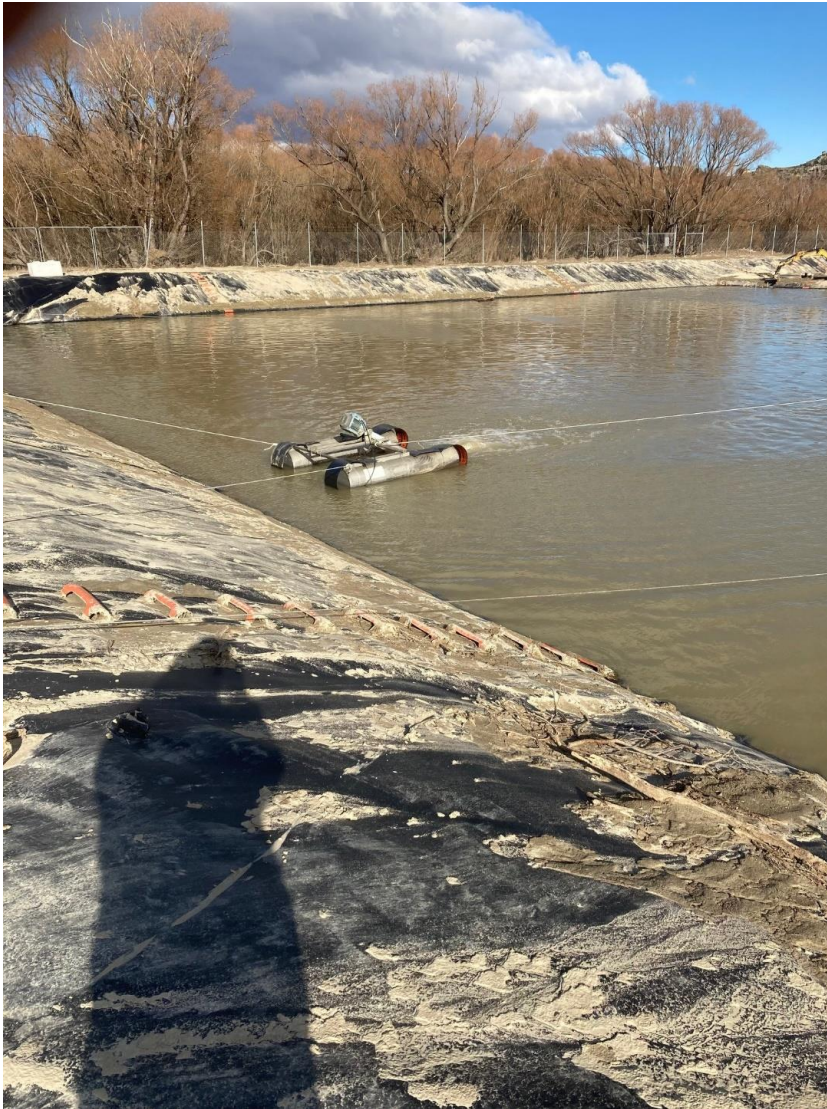
Aerator installed and running
