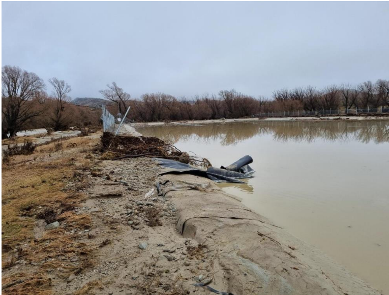
Debris around pond 1, damage to security fence and pond liner visible
