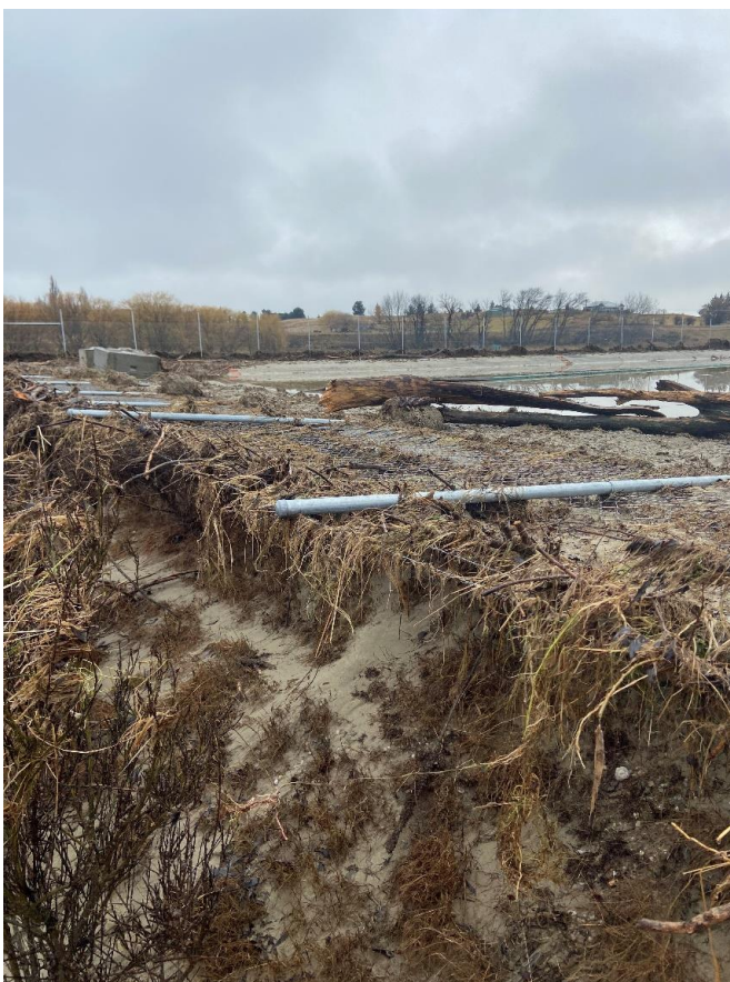
Debris around pond 2, damage to security fence and pond embankment
