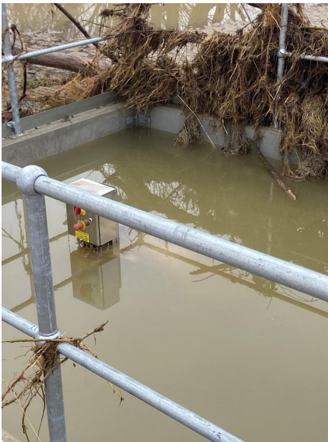
Screen chamber flooded
