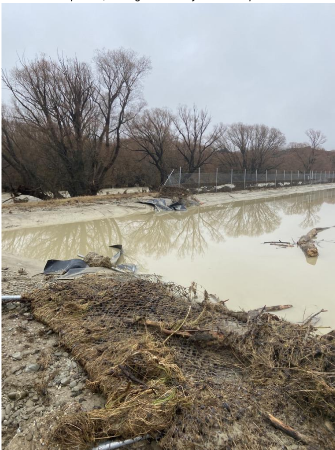
Debris around pond 1, damage to security fence and pond liner visible
