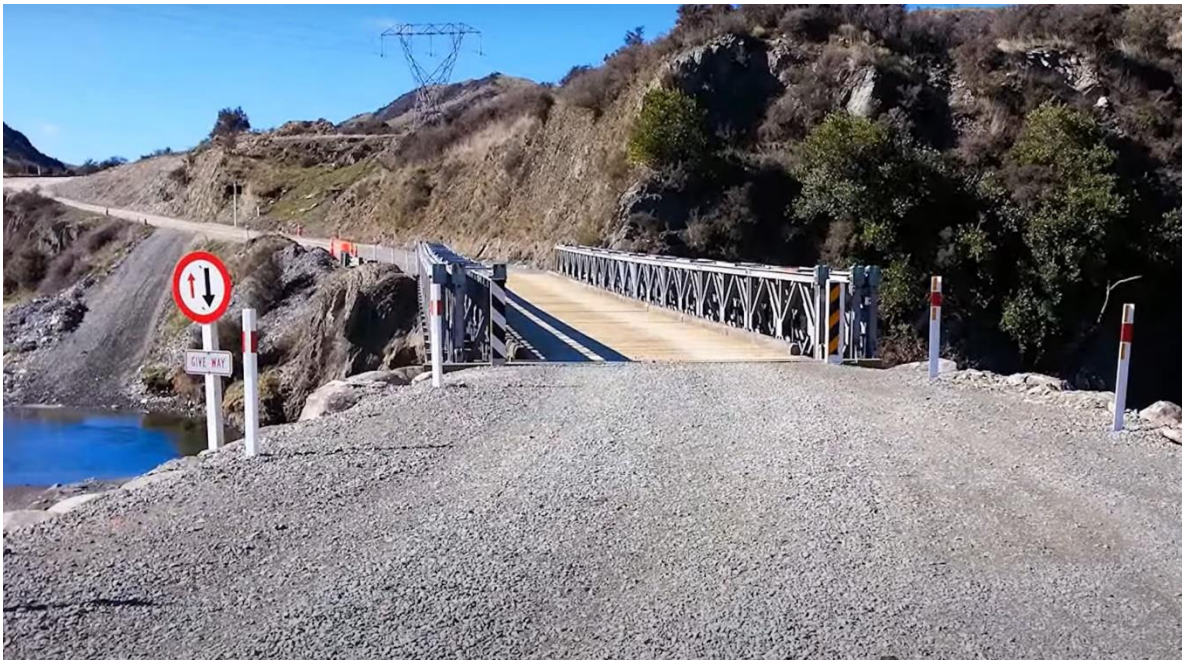
Figure 2: Bailey bridge example
