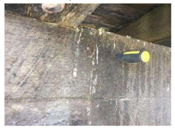
Figure 3 - Deterioration of pilecap beams
