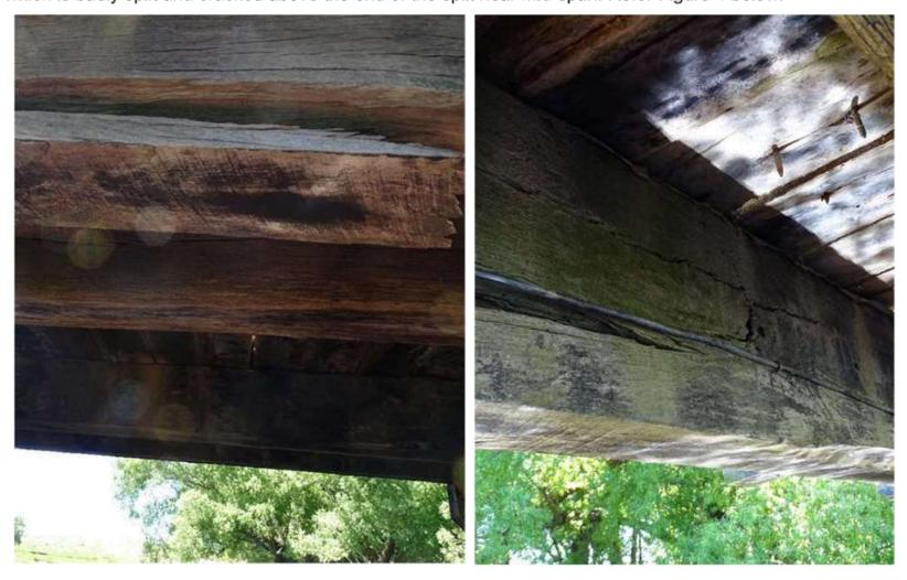
Figure 4 – Split in bottom of longitudinal beam with vertical crack at end of split
