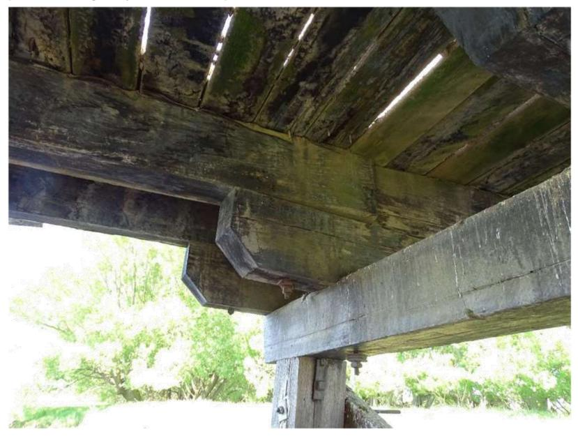
Figure 2 – Pilecap and corbel arrangement
