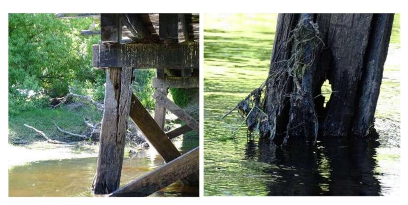
Figure 3 – Typical pile deterioration
