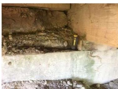
Figure 2 - Deterioration of northern abutment beam
