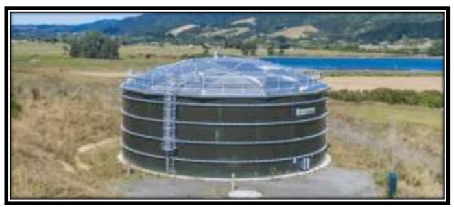
Figure 3 - Example of new bolted steel tank with domed roof.
