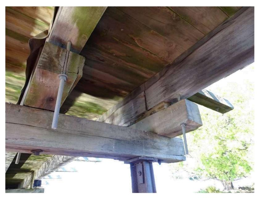
Figure 3 – Additional softwood timber packers installed between the longitudinal beams and the corbels
