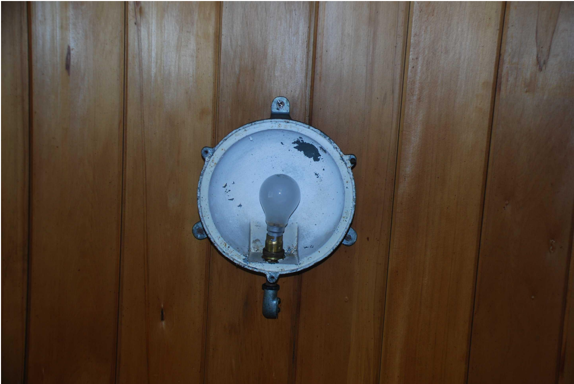
Figure 37 Steel bulkhead light fitting.
