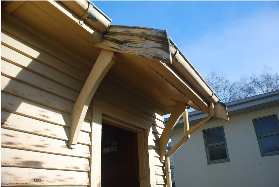
Figure 27 The canopy roof over the entrance door supported on painted timber brackets.
