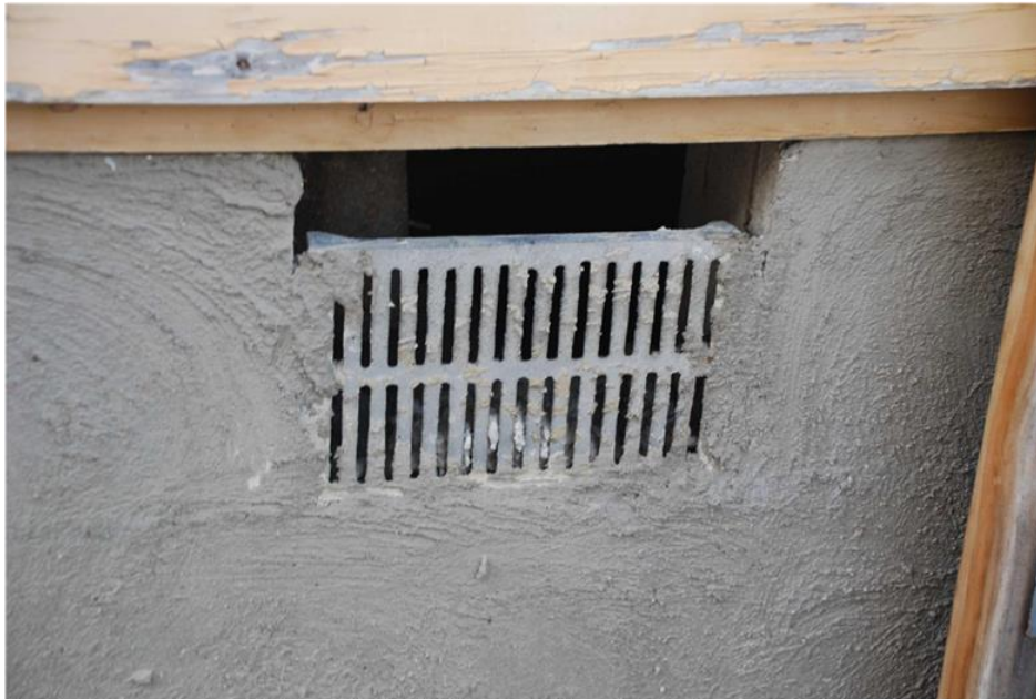
Figure 39 Rendered plinth and airbrick likely to date from about 2003.
