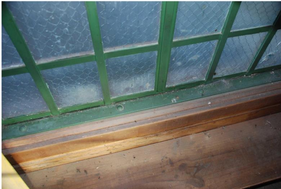
Figure 24 The interior of one of the two cell windows showing how the window is bolted into the framing.
