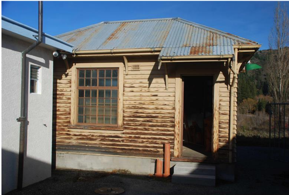
Figure 16 The front elevation with galvanised steel clad hipped roof and projecting canopy over the entrance door; painted, timber shiplap weatherboards; galvanised steel rainwater fittings; eaves brackets; and large, rectangular cell window of galvanised steel with fluted and wired glass. The entrance door leads to a lobby running the depth of the main building.
