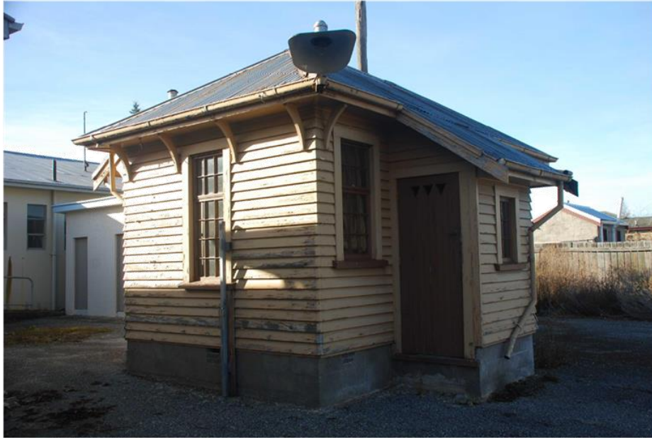
Figure 17 The side and part rear elevation. The left and centre windows light the lobby and the lean-to projection has a small rear window and vented timber door. The lean-to which provided a WC is only accessible from the exterior of the building.
