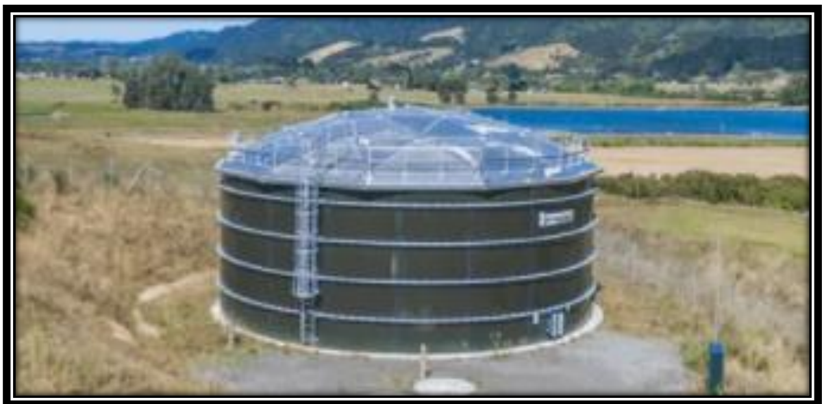
Figure 2 – Example of new bolted steel tank with domed roof.
